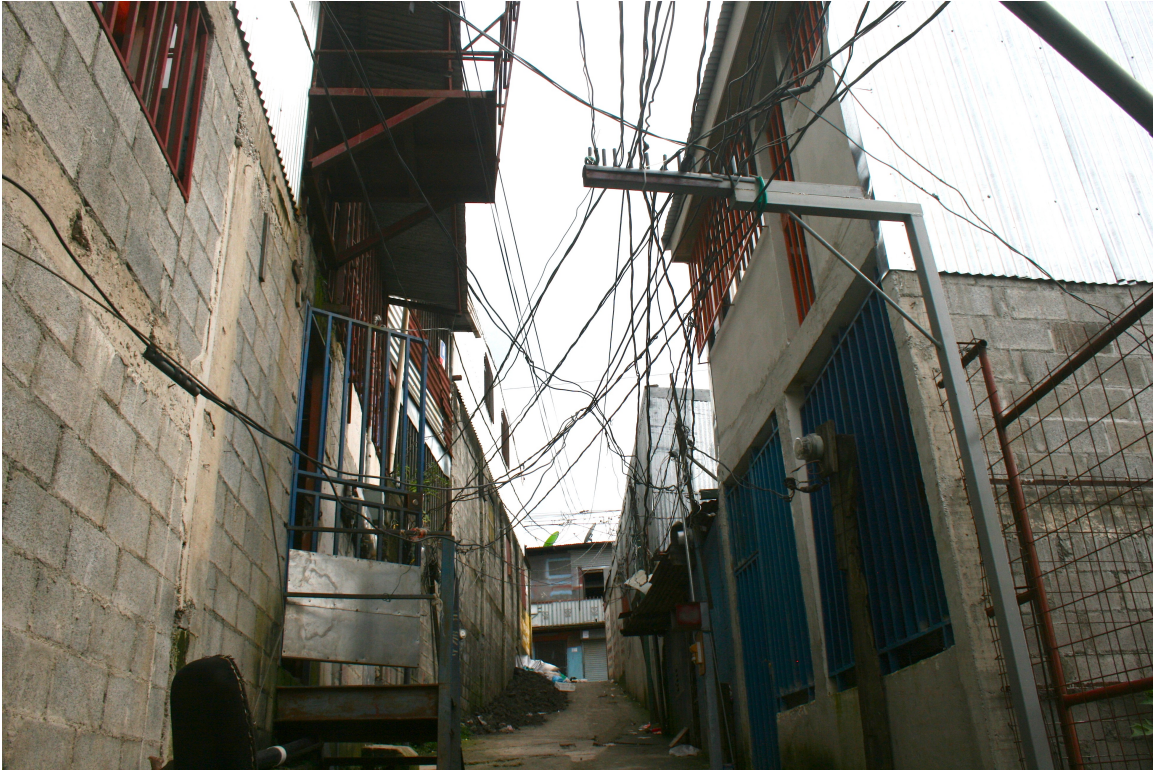
Figure 3. Self-provided electricity. Illegally extending the formal infrastructure from the main road allows these residents to eventually negotiate with the government for the provision of safer connections. This particular infrastructure in Calle Fildadelfia was recently replaced by the Compañía Nacional de Fuerza y Luz who also provided each household with their own electrical meter.
